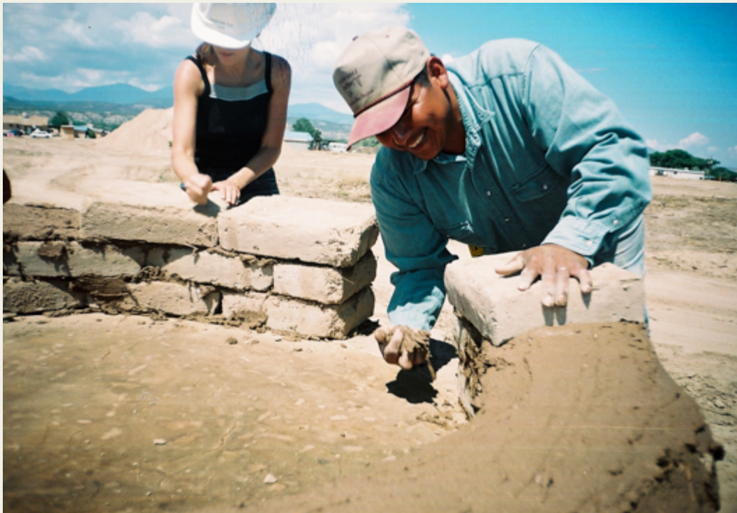
Hand shaping adobe walls in Ohkay Owingeh Pueblo.
